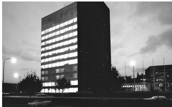
The East Wing after completion, 1976.
